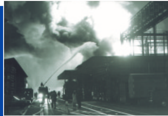
Sandoz warehouse fire, 1986
